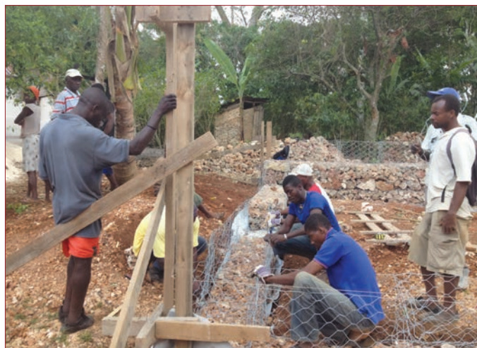
House building using rock-filled gabion cages in Lamontagne
